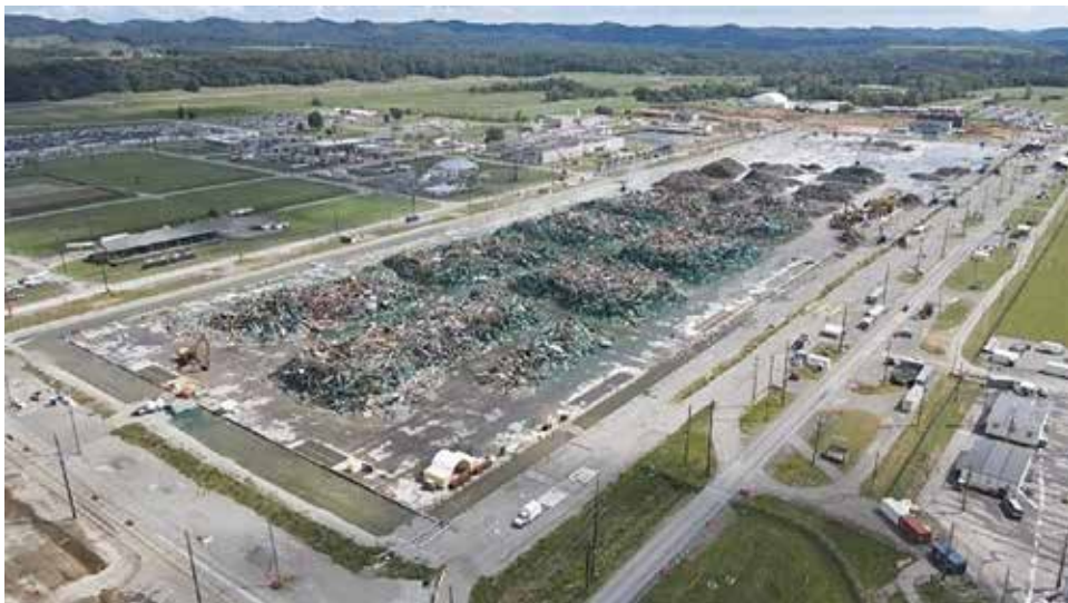
An aerial view of the X-326 uranium process building site following demolition of the Ohio facility earlier this year. The debris will be downsized before compaction and disposal.
