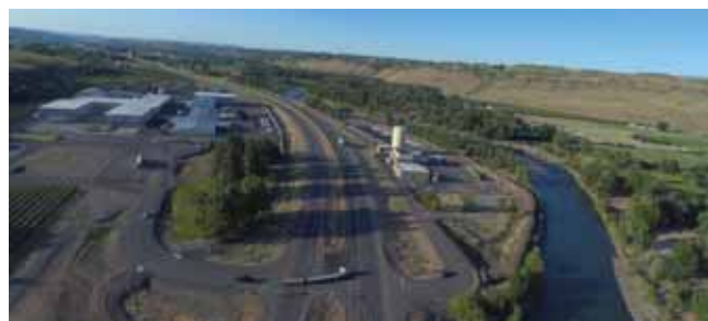
Aerial view of State Route 12 Low Road intersection after completed project. Note: This commercial motor vehicle with double trailers is passing through the intersection into the acceleration lane without stopping in median where it would have blocked the entire westbound freeway.
