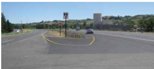
Eastbound State Route 12 Low Road intersection after the acceleration lane was added. Note: The white car closest to the photographer is using the acceleration lane.
