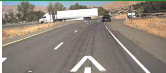
A commercial motor vehicle blocking the intersection and westbound lanes of State Route 12 at Low Road prior to intersection redesign. Note: The black pickup is swerving to shoulder to avoid collision.
