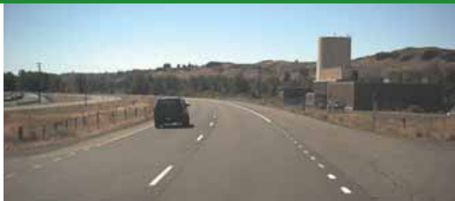
Eastbound State Route 12 at Low Road intersection prior to improvement.
