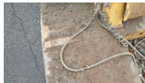
Improper repair to air line on trailer. Photo by Inspector Rod Dykeman, Nova Scotia, Canada.
