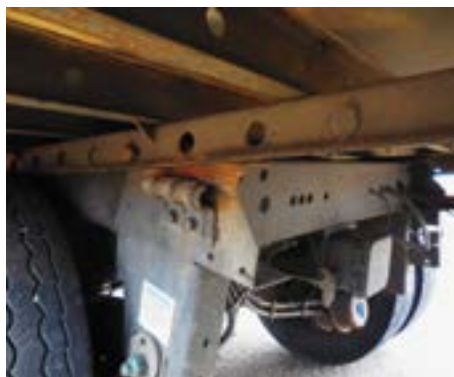
Detached slider guide, broken control arm. Photo by John Watkins.
