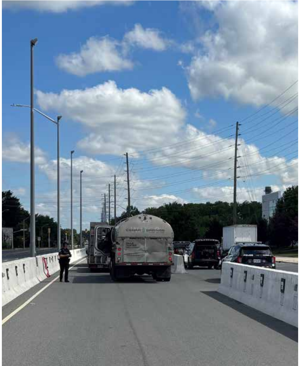
The Region of Halton inspection lay-by lane on Steeles Avenue in the town of Halton Hills.
