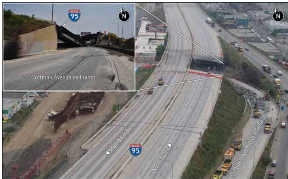
The northbound view of I-95 crash location with collapsed section, from the "Combination Vehicle Rollover, Fire, and I-95 Overpass Collapse" report.
